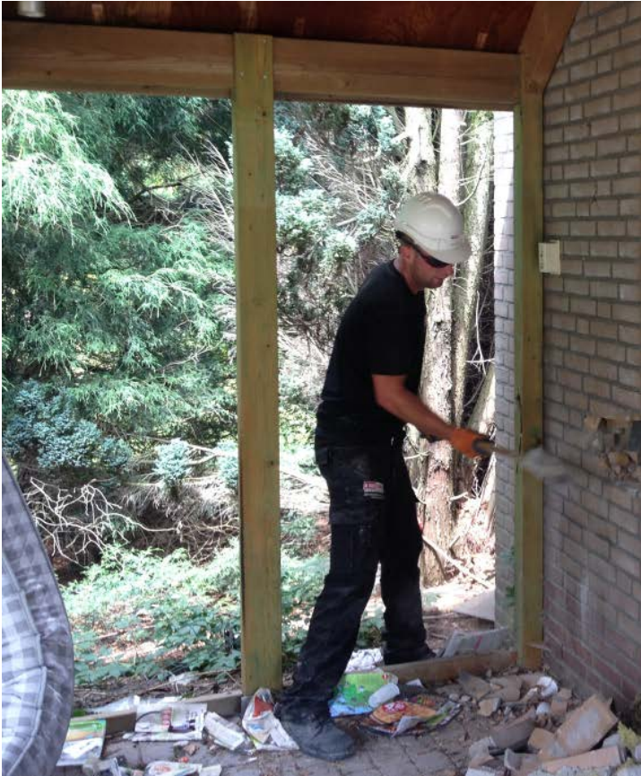
Handmatig slopen (strippen)
